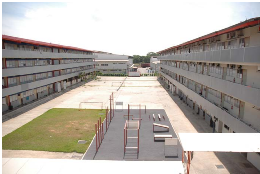
Figure 1 – Exercise facilities situated between two dormitory blocks at Tuas Dormitory
